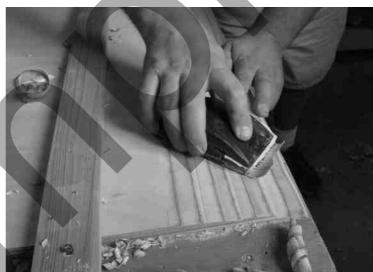
Finished scarfs will have neat, parallel plywood glue lines. The glue lines are a big help in cutting uniform scarf joints.
